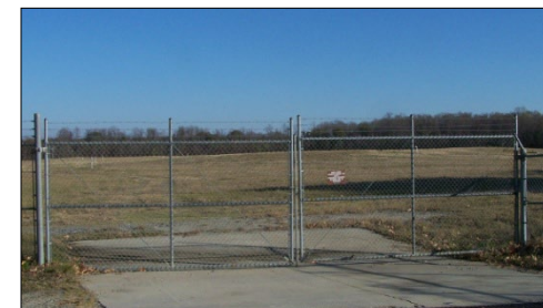
LF004 LUC (Fence and Locked Gate)
