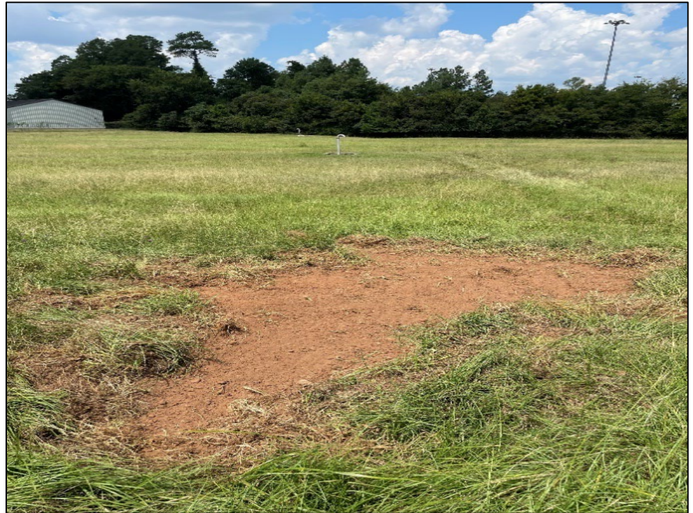
Repair of Vegetative Cap
