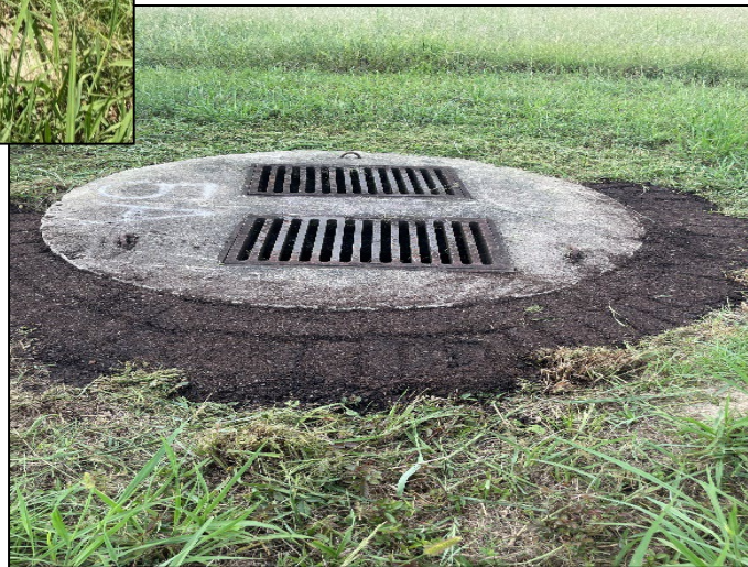
Erosion Repair at Inlet
