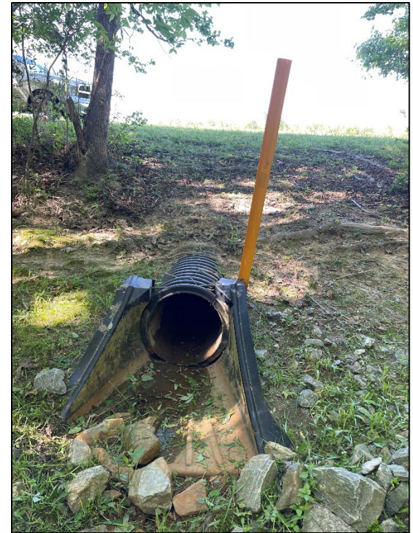
Clearing and Grubbing at Outlet
