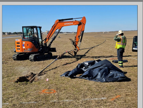
Installation of a horizontal well at SWMU 60.
